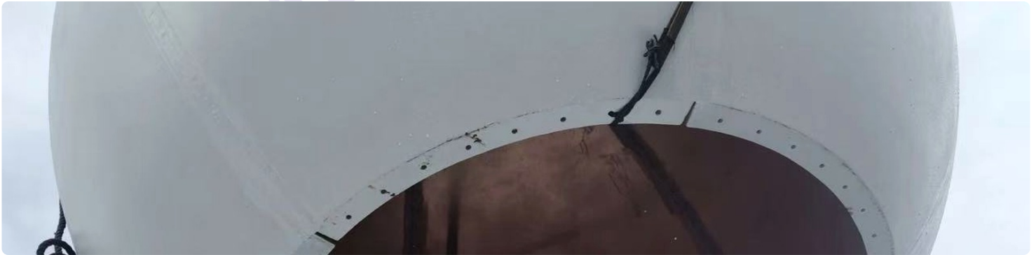
Photo: White multi-panel sphere under crane lift; bolted base flange ring visible. No customer or site named.
